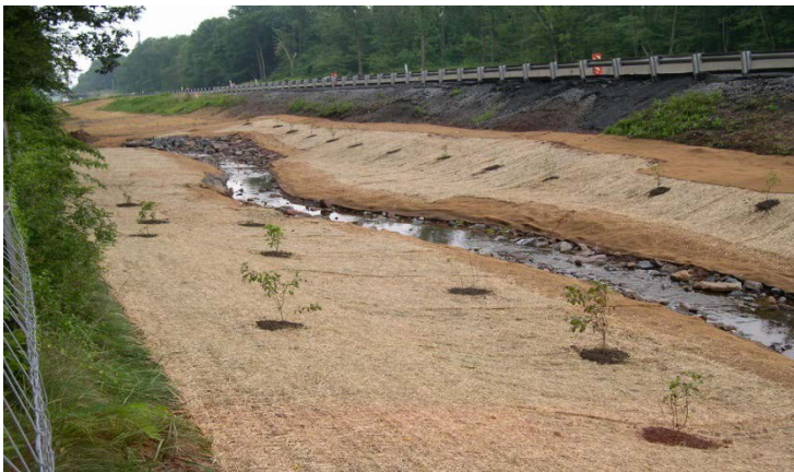
Figure 1: Streambank Rehabilitation Project
